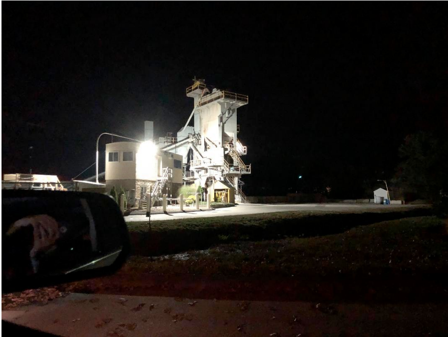
Amherst batch plant, October 24, 2019, 10:40 PM
