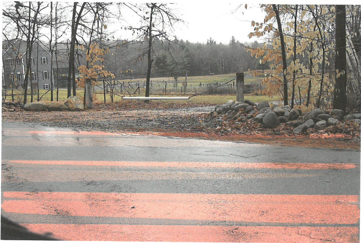
Photos of unpermitted access road at 834 Mason Rd. taken on 3/25/2016 by John Shepardson.
