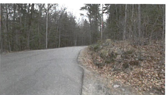
Isaac Frye looking north
