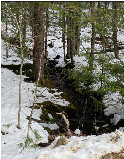
Roadside view of a stream flowing under Duggin Road.
